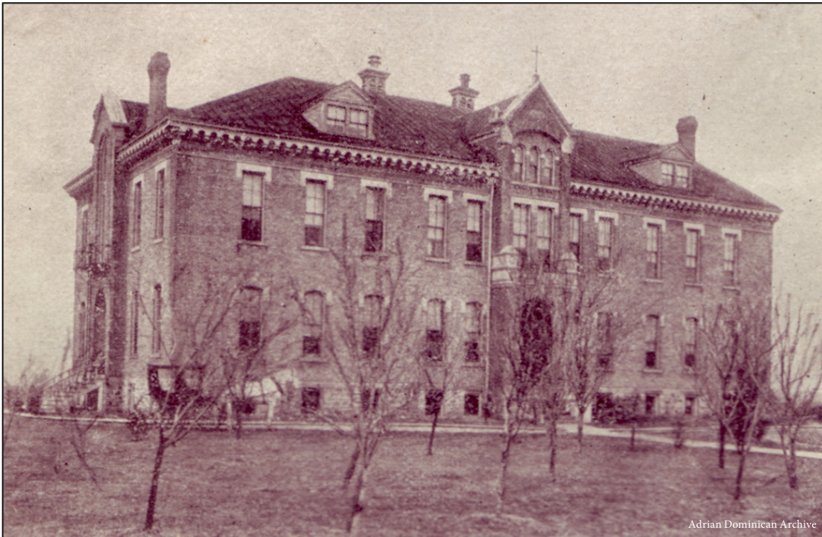
The “red brick building,” constructed in 1886, became the home of St. Joseph Academy and site of the motherhouse of the Adrian Dominican Sisters.
